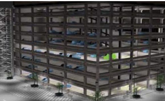
As visitors exit, luminaires on each level illuminate to full power.
